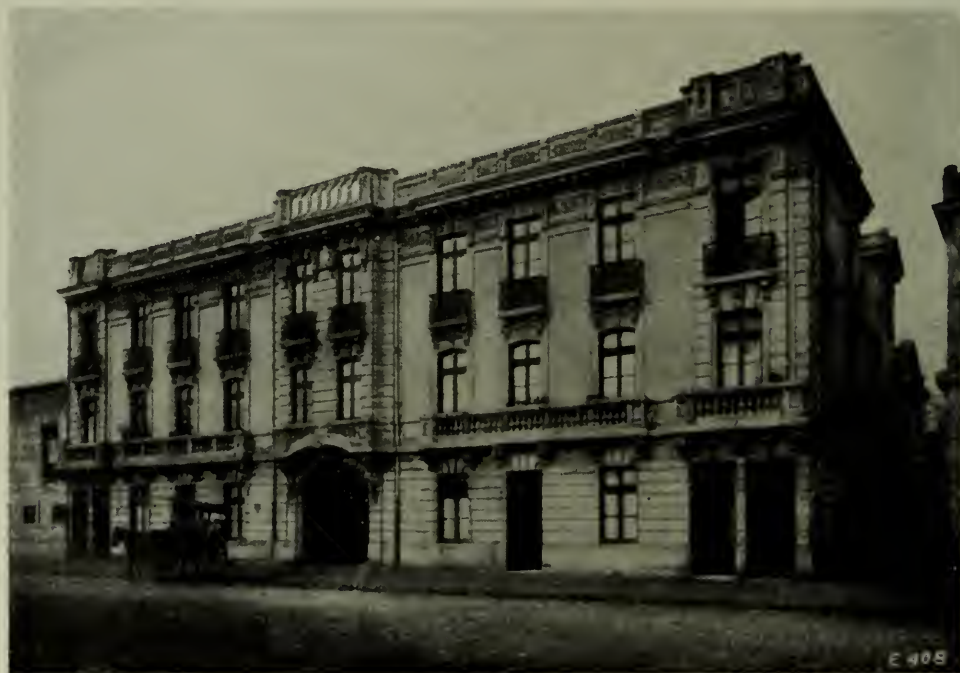
BUILDING IN CHACABUCO STREET, VALPARAISO. (See page 255.)
